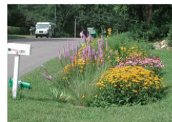
Figure 8.3 A bioswale in a residential neighborhood in Lake County, Illinois. Photo Source: Lake County, Illinois
