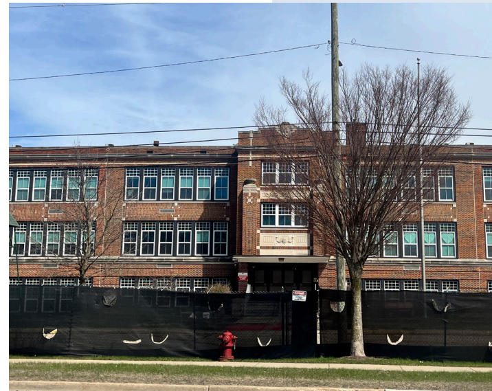
Figure 5.4 Roosevelt Elementary School as pictured in April 2025.
