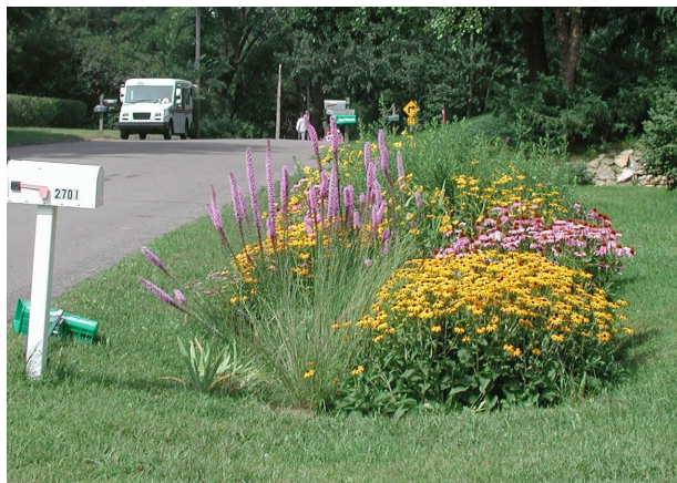
Figure 8.3 A bioswale in a residential neighborhood in Lake County, Illinois.
