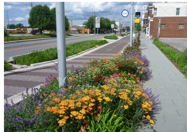
Figure 8.4 Bioswales can also be used to divert stormwater in commercial or public areas while beautifying the corridor, as was accomplished by the Indianapolis Cultural Trail.
