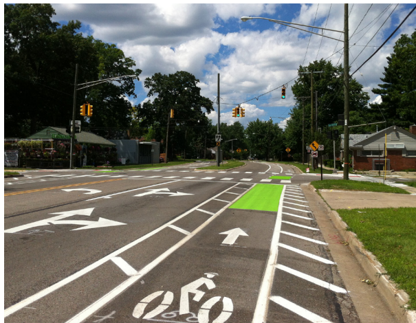
Figure 6.4 The Complete Streets project on Livernois between 8 and 9 Mile Roads funded by TAP included bike lanes among other improvements.
