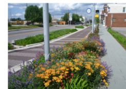
Figure 8.4 Bioswales can also be used to divert stormwater in commercial or public areas while beautifying the corridor, as was accomplished by the Indianapolis Cultural Trail. Photo Source: Indianapolis Cultural Trail
