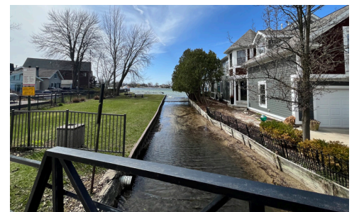
Figure 2.3 The Willow Beach Street Swim Site located on Willow Beach Street north of Kenrick Street is one of three public access points to the waterfront. These sites offer very little frontage along the water, as demonstrated in the picture above.
